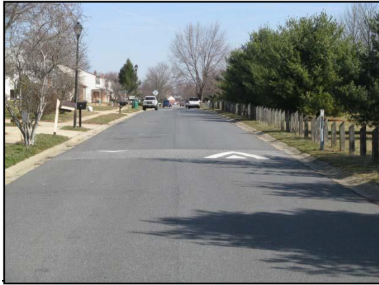
SPEED HUMP (Valley Forge Road)
