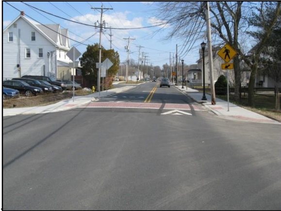
RAISED CROSSWALK (Old Lancaster Pike)
