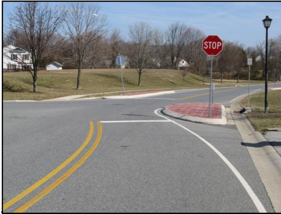
REALIGNED INTERSECTION (Old Forge Road)
