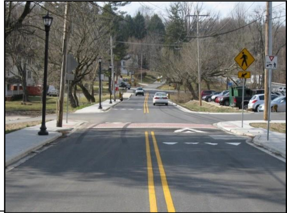
RAISED CROSSWALK (Old Lancaster Pike)
