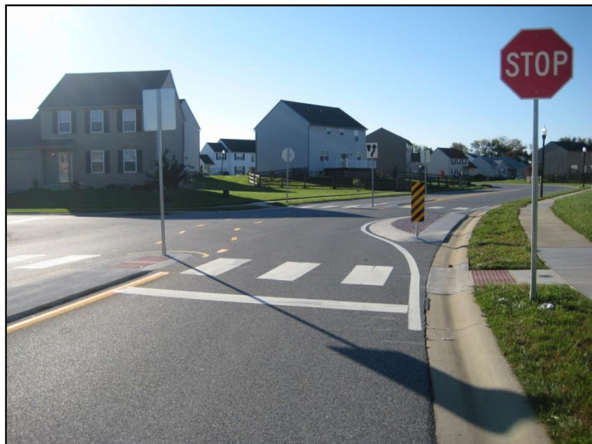
CROSSWALK AND SIDE ISLAND STRIPING ON A SUBDIVISION STREET
